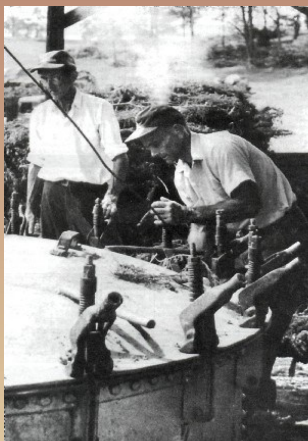
Fastening the clips on a Wormseed Kettle. http://www.farmcollector.com .
